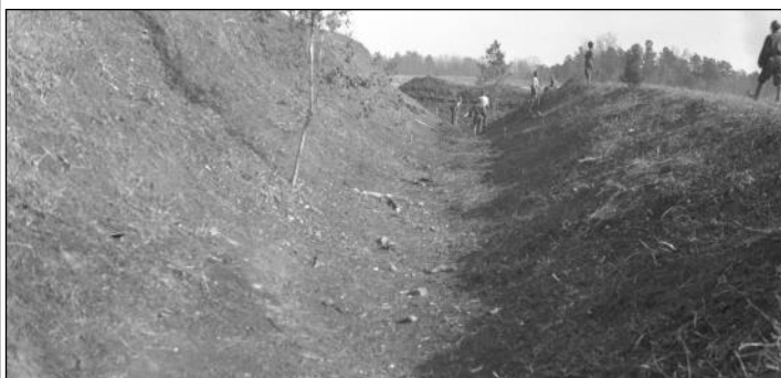
Restoration work at Ft. Hoke, 1930s (RNBP archives)
