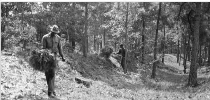
Checking erosion on earthworks, 1936 (RNBP archives)
