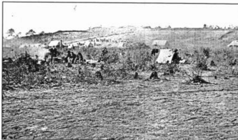
The cameraman stood on what now is RBA property when he took this photograph of Fort Harrison in 1865. The wall of the fort is visible on the skyline. The swale in the middle distance is our northern boundary. The photograph under the masthead (top) shows the "Great Traverse" and the southeastern face of Fort Harrison.
